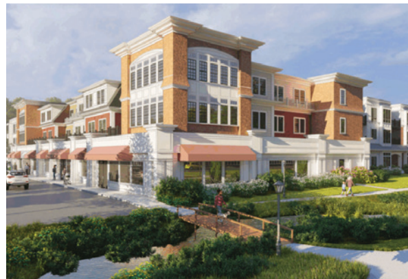
The Block at 22 Everett Street in Westwood, MA, developed by Giorgio Petruzzello of Supreme Development
